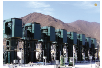
Shuqaiq IWPP Motors Ordered In November, we won our largest electric motor order to date for the USD 1.9 billion Shuqaiq independent water and power projects in Saudi Arabia. The USD 12 million order from Water & Electricity L.L.C. includes a total of 235 motors in 34 different models—including 13.2 kV high-voltage units—that will pump over 212,000 cubic meters of potable water daily when completed in 2009.
