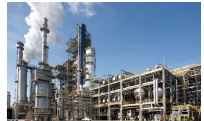
#2 HOU plant completion
