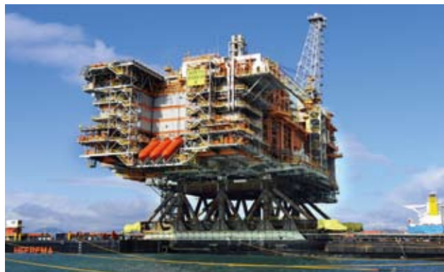
North Rankin 2 topsides delivered The North Rankin 2 topsides were ordered by Woodside Energy of Australia for the North Rankin 2 (NR2) project, a project designed to recover the remaining low-pressure gas from the North Rankin and Pegasus gas fields off the northwest coast of Western Australia. Following load out in December 2011, the 29,000-ton topsides sailed for Australia in January 2012.
