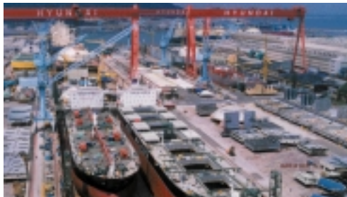
Dry Dock #2 with a capacity of 700,000 DWT
