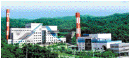
Sunghnam Municipal Waste Incineration Plant, Korea
