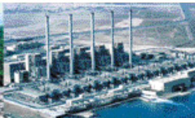
Al-khobar PH-II Desalination & Power Plant, Saudi Arabia
